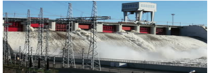
Fig 3: A Dam with Hydro power station.
