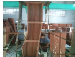
Fig 18. Failure mode of CFS-C-1-S-2
